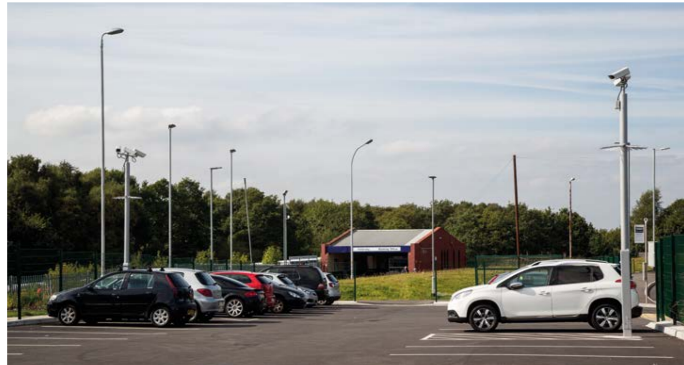
Figure 19: New car park for railway station
