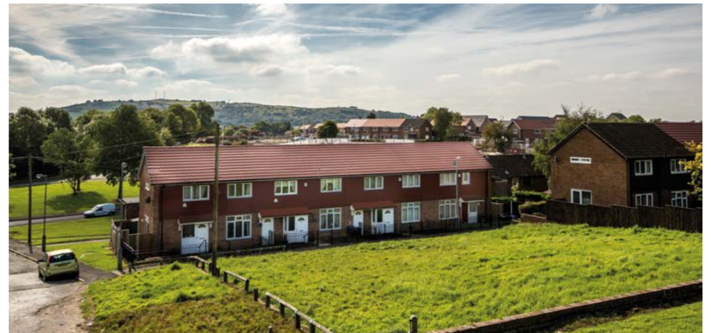
Figure 16: Typical quality of public realm in Hattersley
