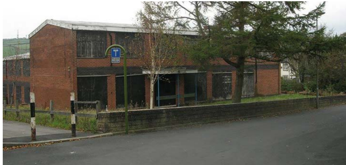
Figure 22: typical dereliction in Hattersley before regeneration process
