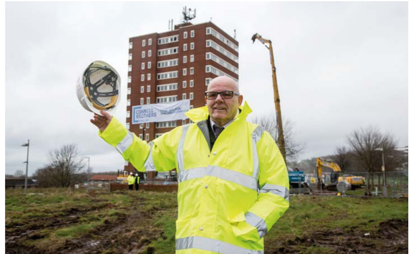
Figure 11: Demolition of the last tower block, Tameside Court, in 2017
